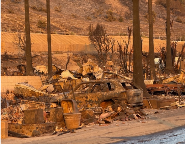
Devastation along PCH.
